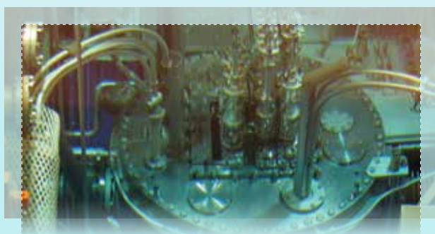
SAFARI-1 reactor core vessel and rigs for irradiation procedures
